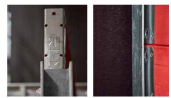
The decks or panels are inserted into the I girder from above, where they then form a stable wall of up to 5 cm in thickness.
